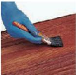
Starting at the top of the jamb, apply stain with a 3" to 4" soft bristle brush or rag. Apply enough stain to fill the jamb grain. (Refer to the jamb staining diagram.)
