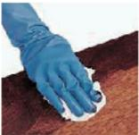
With a clean, lint-free 24" x 24" cloth or soft bristle brush, softly wipe the surface until you reach your desired tone. **TIP:** When the rag becomes saturated with stain, re-fold to work with a less-saturated section. Be sure to use the same rag for the whole jamb. If using a brush, dab excess stain from brush into a clean rag.
