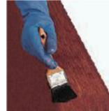
Application of a good exterior UV-inhibitor polyurethane top coat.
